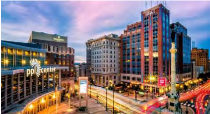
Allentown's PPL Center and City Center Projects (PA)
