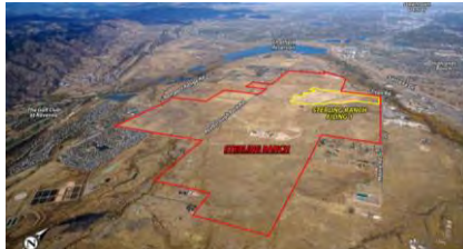
Dominion Water & Sanitation District Douglas County
